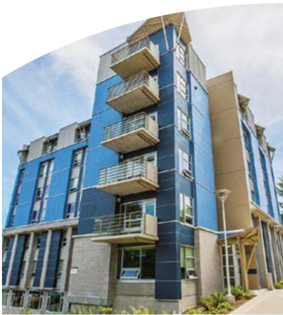
Live in one of our nineteen residence buildings on campus.
